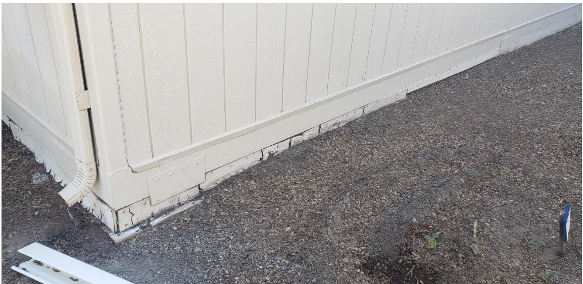
Repair and Replace Skirting
