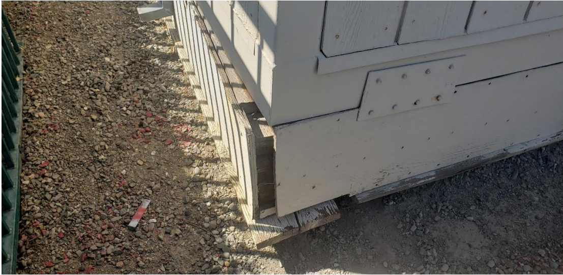
Repair and Replace Skirting
