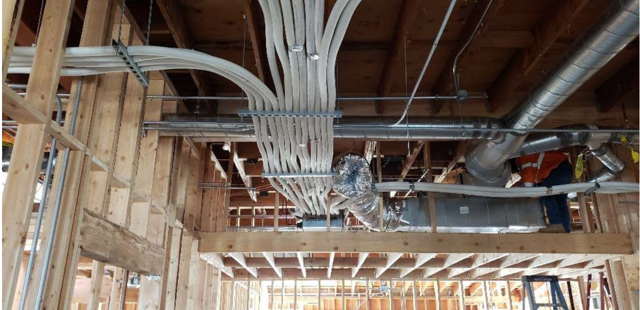
Line Sets for HVAC Units
