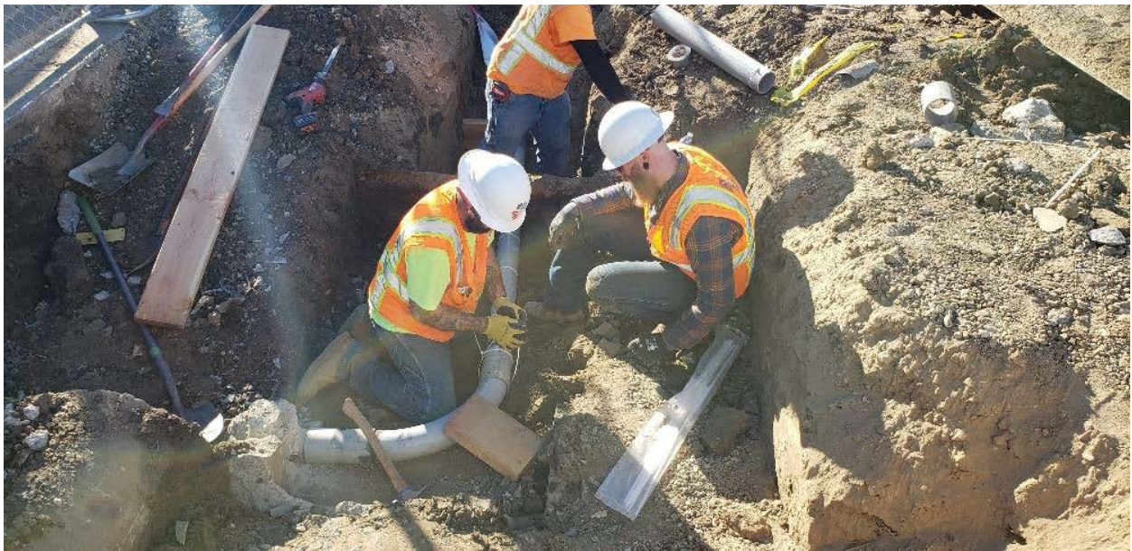
Sweep connection work to new PG&E service vault
