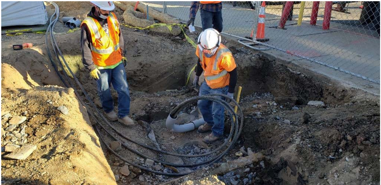
Power transition work from exiting service to new
