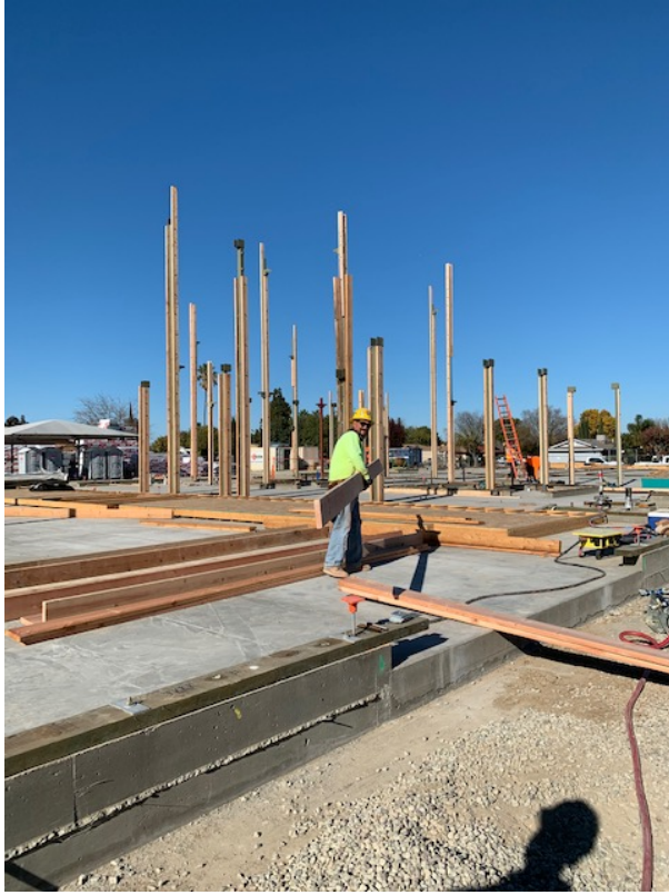
Steel columns have now been erected.
